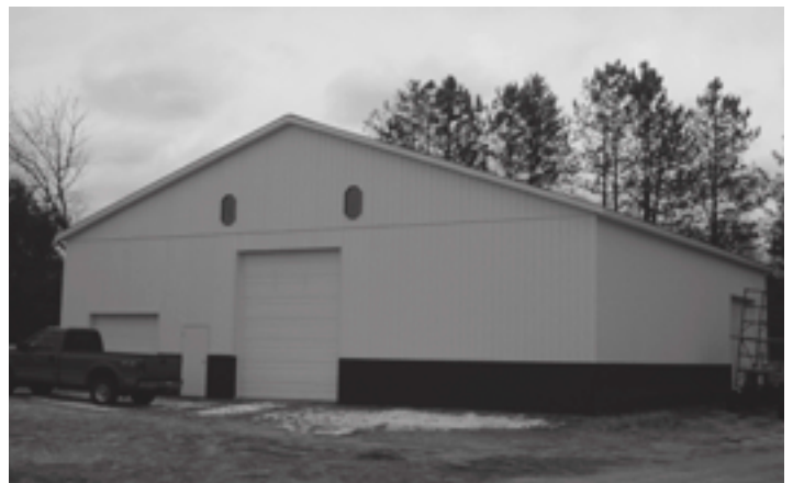
The new storage barn at the Society's Lawton, Michigan, retreat center is already standing and functional. (PHOTO COURTESY OF BR. JOSHUA CASWELL, SSJC)
